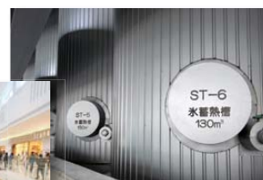
Ice thermal storage systems use off-peak power to accumulate ice in the thermal storage layer that is used for cooling during the day.
