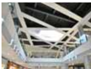
Ceiling with higher aseismic capacity
