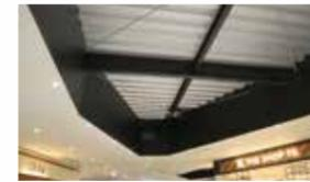
We design the ceilings of atrium spaces to minimize secondary damage from falling objects by reducing the weight per unit area.
