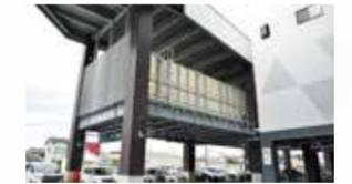
Important equipment, including power facilities, are installed in high locations that are not affected to avoid flooding from tsunamis or other water damage.
