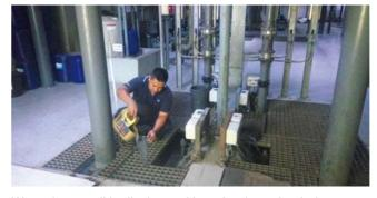
Water from mall is discharged into the river after being treated by septic tank equipment using bacteria. Mall conduct water quality inspection once a month and have confirmed that local effluent standard which is said to be stricter than Japanese standards is cleared.
