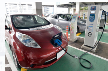
EV charging station (AEON MALL Zama (Kanagawa Prefecture))
