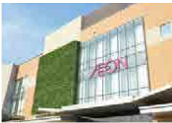
Planting on wall surface
