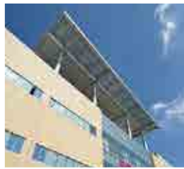
Installing solar power facilities
