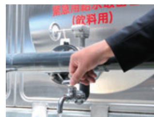
Faucet for emergency water access
