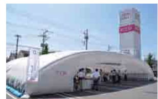
The balloon shelter serves as an evacuation site during emergencies.
