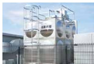
▲ Elevated water tank installed on the roof in case of a large tsunami (AEON MALL Sakai Teppouchu)
