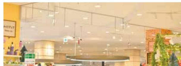
New malls opened after the Great East Japan Earthquake have adopted construction methods to increase aseismic performance at major points of the ceiling, by using a film-reinforced ceiling or an uncovered ceiling design for main walkways. Water receiving tanks are also constructed anti-seismically and durably to withstand earthquakes of a similar scale to the Great East Japan Earthquake.
