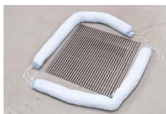
Oil protection wall installed in a garbage storage
